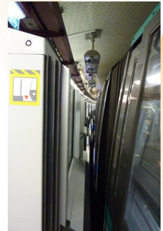
Laser sensors monitoring gaps
